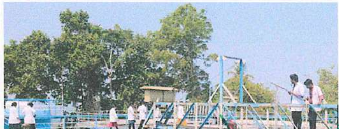
Water treatment plant visit
