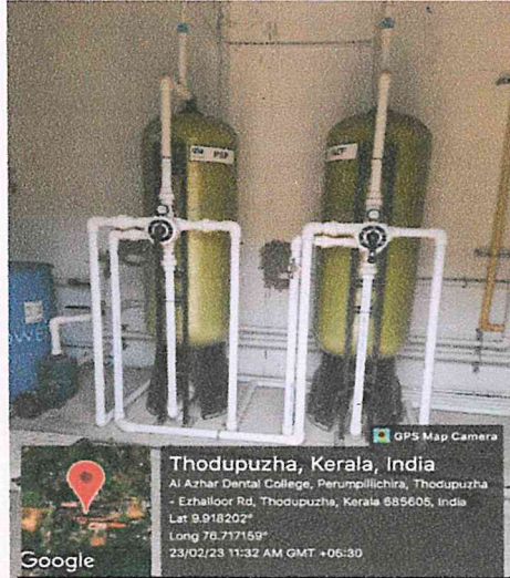
FINAL FILTER WITH CHLORINE DOSING
